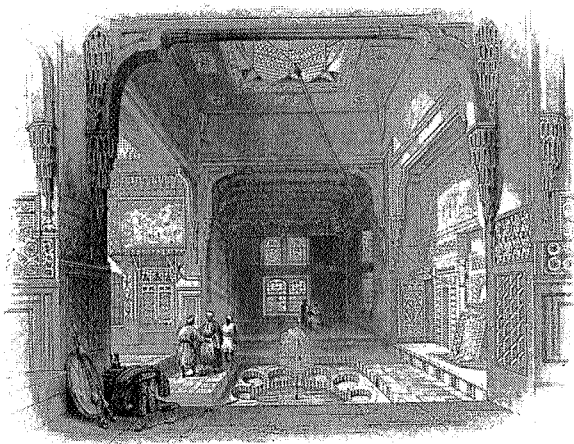
INTERIOR OF A HOUSE
